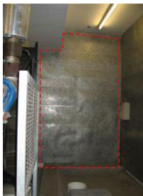
Sound insulation layer on walls
