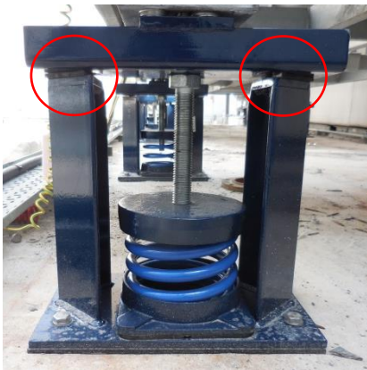
Defective implementation of a vibration isolator
