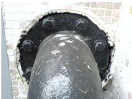
Insertion of Flexible Sleeve at Wall Penetration Locations of Pipes
