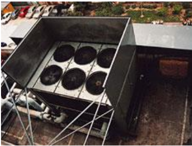
Installation of Noise Barrier
