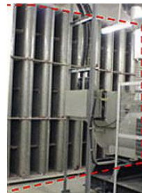
Silencers at air inlet and outlet
