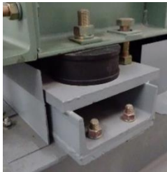
Figure 35 : Anti-vibration pad for Traction Machines
