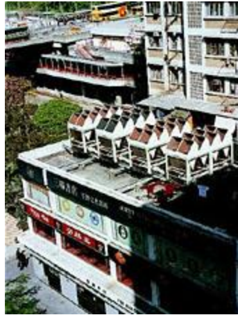
Orientation of Exhaust Outlet Away from Noise Sensitive Receivers
