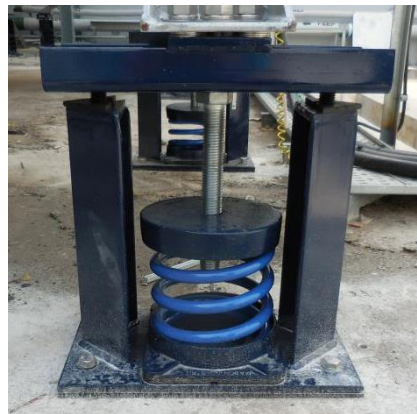
Normal implementation of a vibration isolator
